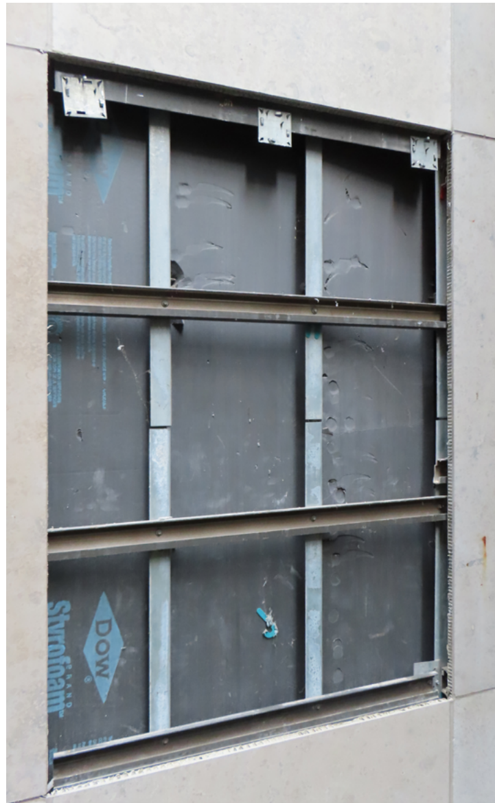
Example of framing that connects stone panels to the building structure.
